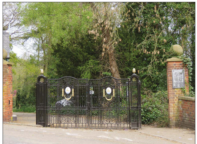
Figure 48: Gates to The Warren and Hartham Common, Port Hill.
