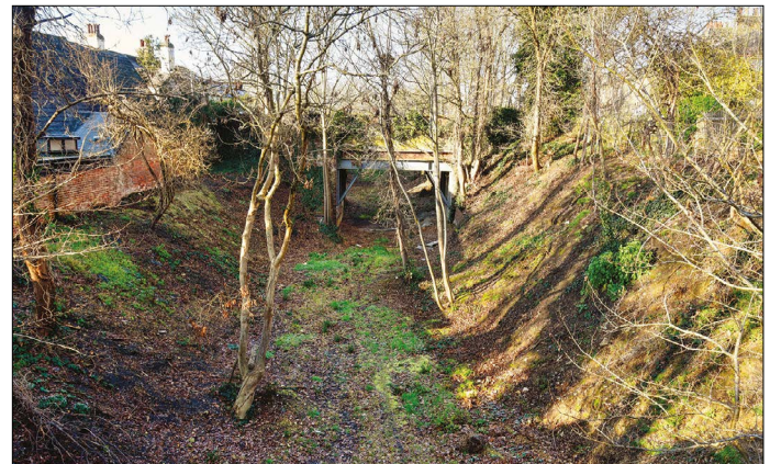
Figure 5: Former Railway Line, looking west.
